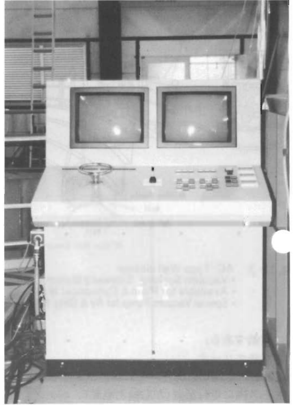
Photo 2 Control Desk for Tank Bottom Cleaner
